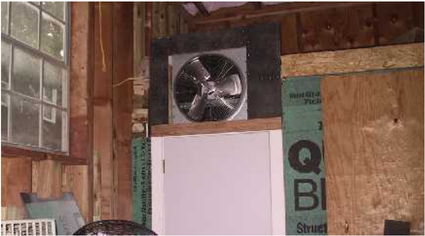
New fan going in. Exit will be a pipe in window.
