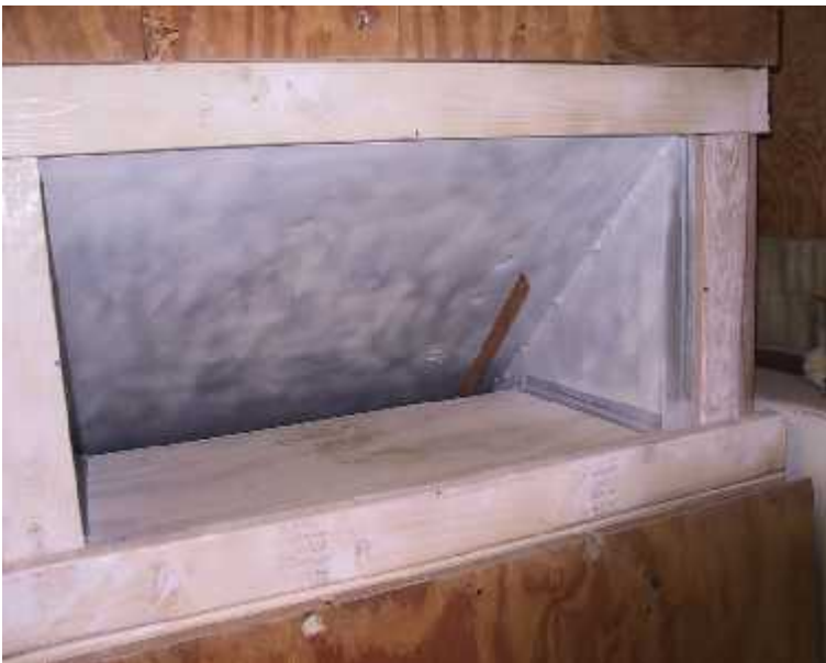
New 'sand' trap up close. About 3 feet wide. 3/8 steel.
